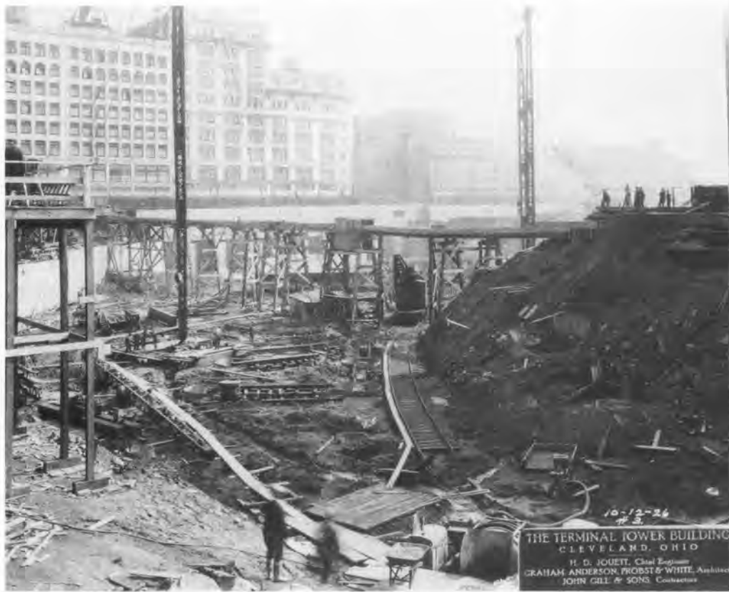
Future site of Higbee's Department Store, October, 1926, after partial excavation and construction of retaining walls along Ontario Street. Excavated material was hauled by train and truck to the west side and to the lakefront, where it was used as fill. CSU Archives.
